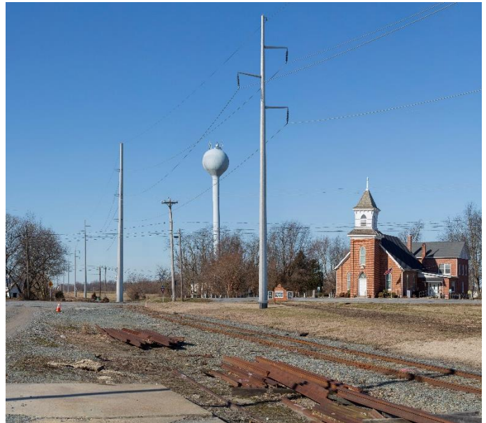
This photo rendering shows what the new galvanized steel poles are expected to look like along the rebuilt transmission line in Kent County.
